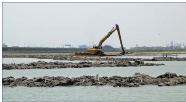
Marsh buggies dig up sediment for terraces in phase 1.
