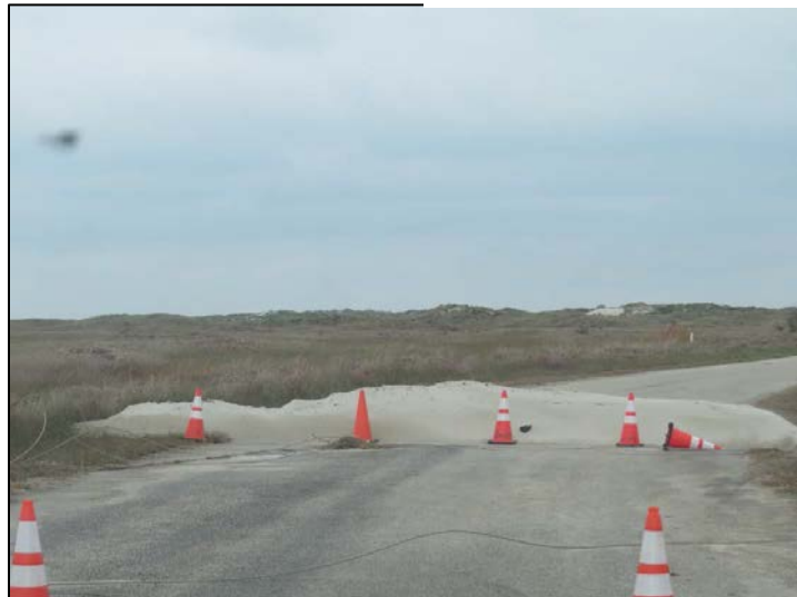
Extensive damage to infrastructure at Mustang Island State Park will take many months to repair before it can reopen to public.
