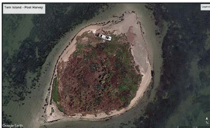
Erosion damage on Tern Island; approximately 15-40 feet of shoreline loss. A floating cabin and debris are visible.
