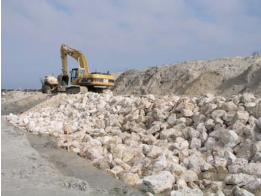
Port Aransas Nature Preserve Shoreline during Construction (Now)
