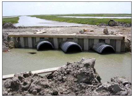
This culvert, installed as part of a Coastal Bend Bays & Estuaries Program project, helps water flow through the wetland, which revives marsh habitat for fish, shrimp and crabs.
