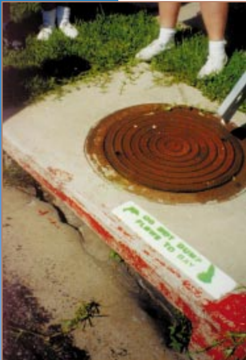
Inlet stencilled with a message to prevent debris from being improperly discarded.
