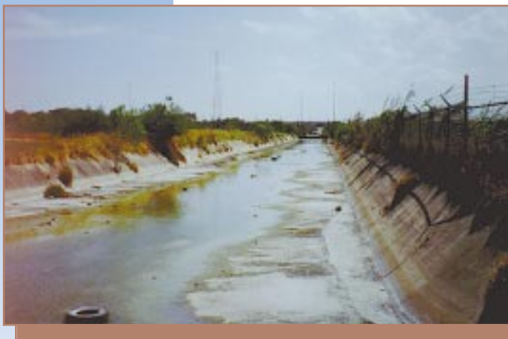
A typical drainage way found in the Coastal Bend designed to drain rain water. These systems not only move the water quickly but pick up pollutants from surrounding property.
