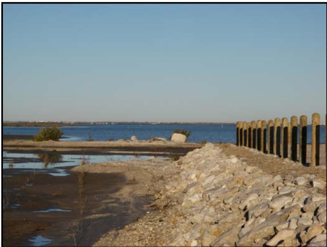
Armor stone placed around edge of parking area
