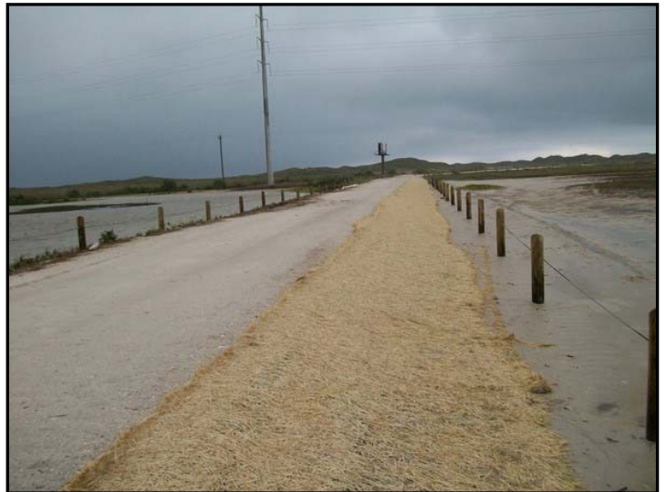
Erosion Blanket installed along edge of new access road
