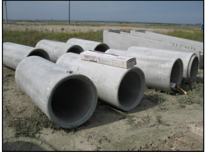
Culverts to be placed along HW 361
