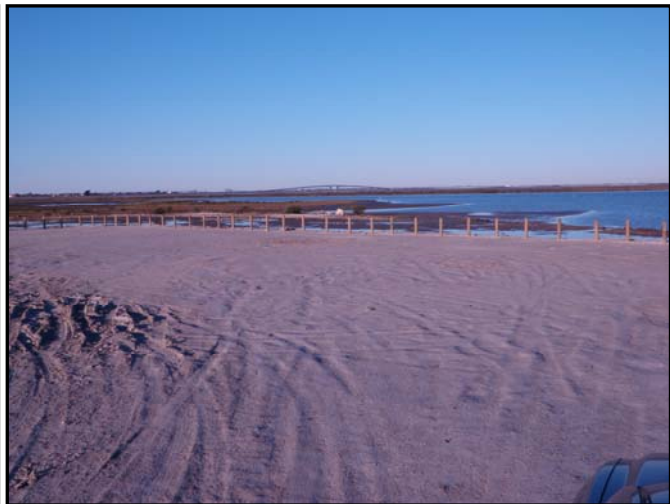
Finished 1/2 acre parking area
