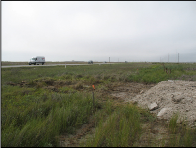
Entrance prior to installation of TxDot permitted access
