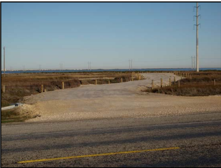
Finished HWY 361 access
