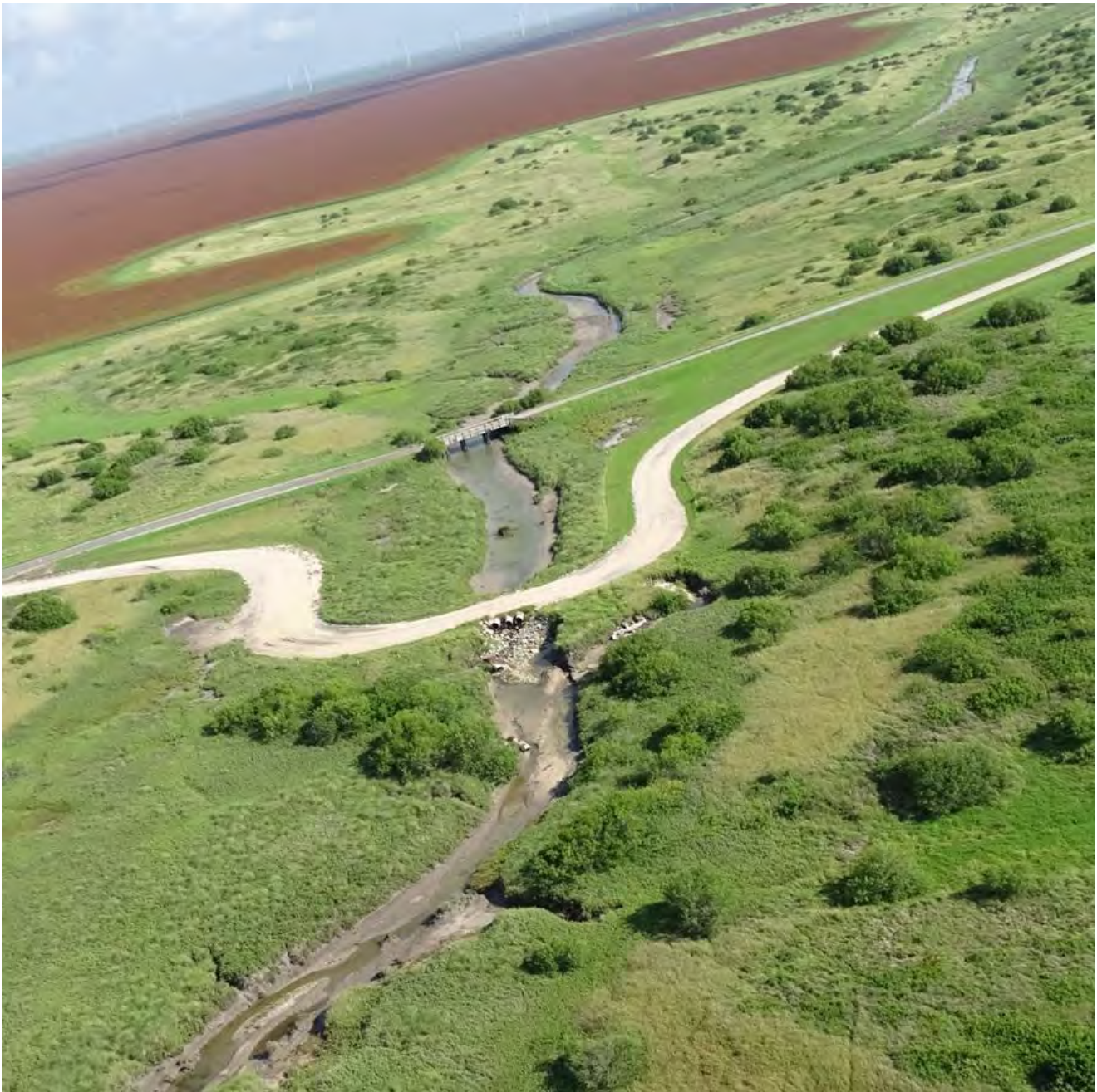
Figure 118 The poorly designed crossing pictured in the foreground is acting as a gradient control structure and is a source of erosive energy evidenced by scoured banks and gully formation. In contrast, the crossing pictured in the background is well designed to allow passage of sediment and water without enhancing the streams erosive energy.
