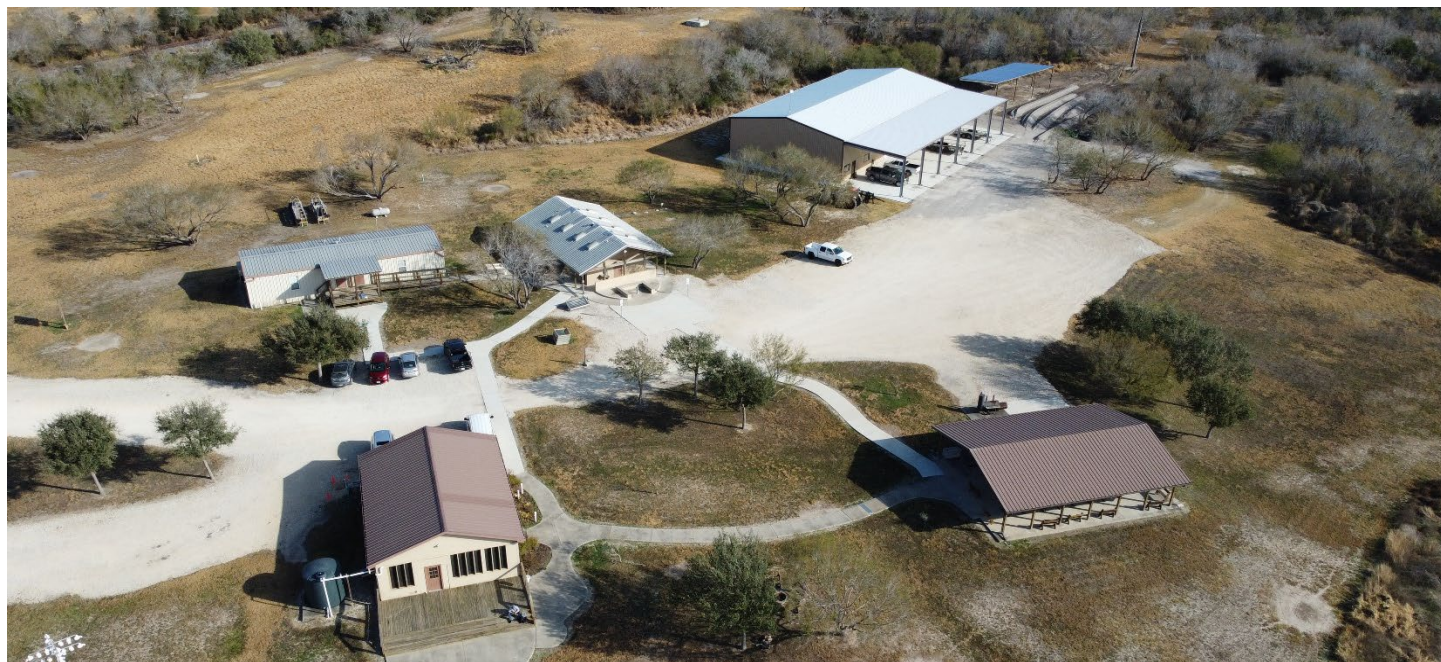
Education Center and Land Conservation Headquarters at Nueces Delta Preserve
