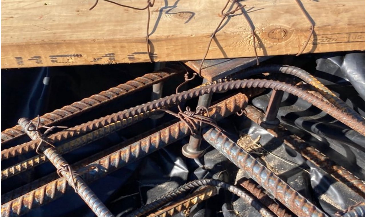
Slab corner weld-plate and rebar installation
