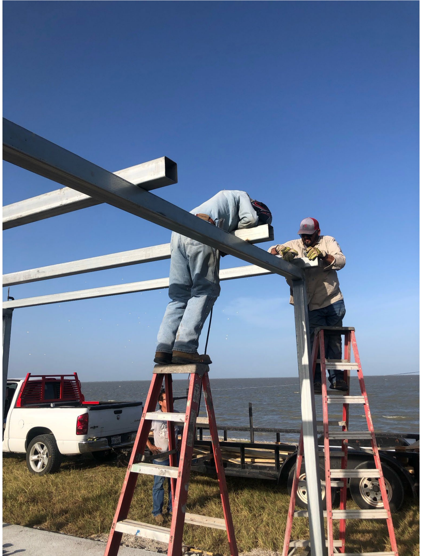
Welding the rafters into place
