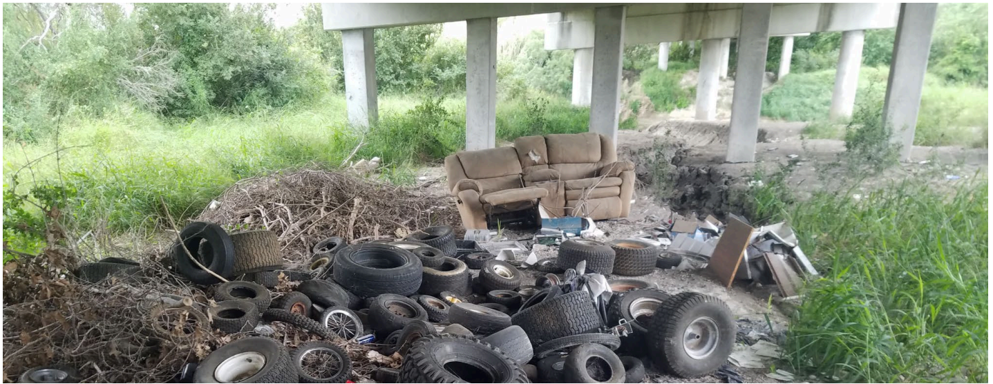
Typical illegal dump site, these items were dumped along Petronila Creek under FM70 and cleaned up by TXDOT.
