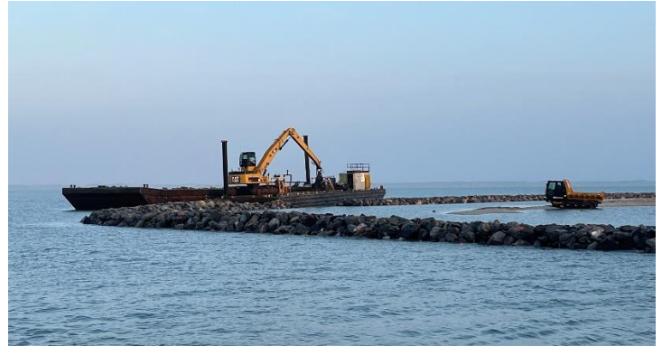
Construction of breakwater from barge and marsh buggy.
