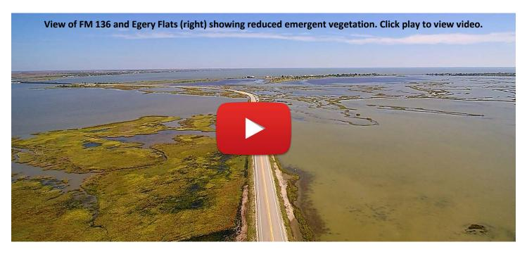
FM 136 was placed across the marsh with only two water exchange points, and while it connected communities and provided public access to the flats, it also limited water flow. Over time the culverts at the water exchange points became clogged and the water flow was restricted enough to impact water quality and habitats, which has resulted in the conversion of over 100 acres of estuarine marsh and vital habitat to open water since the 1950s.
