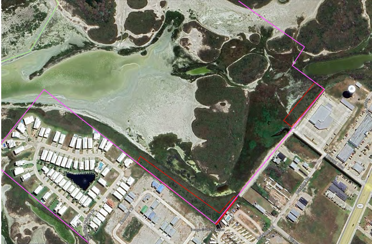
Figure 4. Delineated in red are the 1.3-acre and 0.75-acre areas in the Nature Preserve at Charlie's Pasture where Brazilian peppertree was shredded. The City will install additional anti-vehicular fencing in this area (delineated in pink). The City will also hire a contractor to spray herbicide on the regrowth of Brazilian peppertree.
