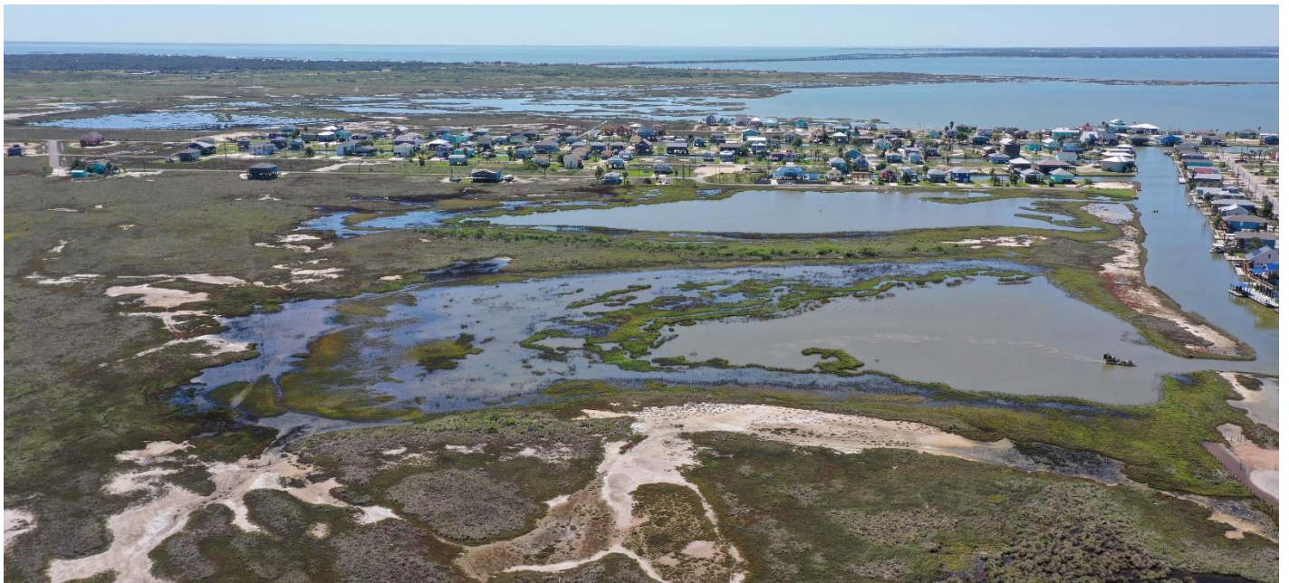
View of Holiday Beach community and surrounding wetlands that benefited from debris removal.
