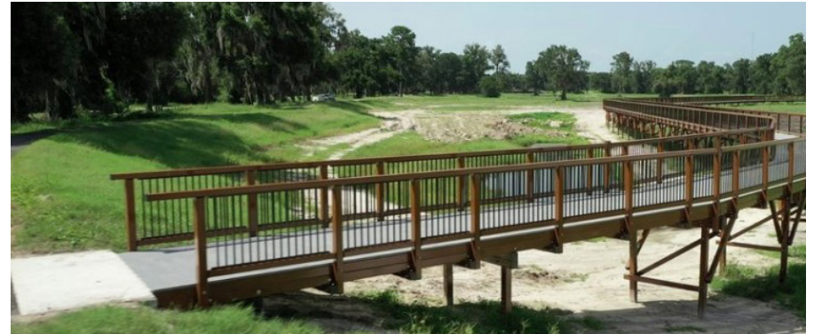
Fiber Reinforced Polymer (FRP) Boardwalk
