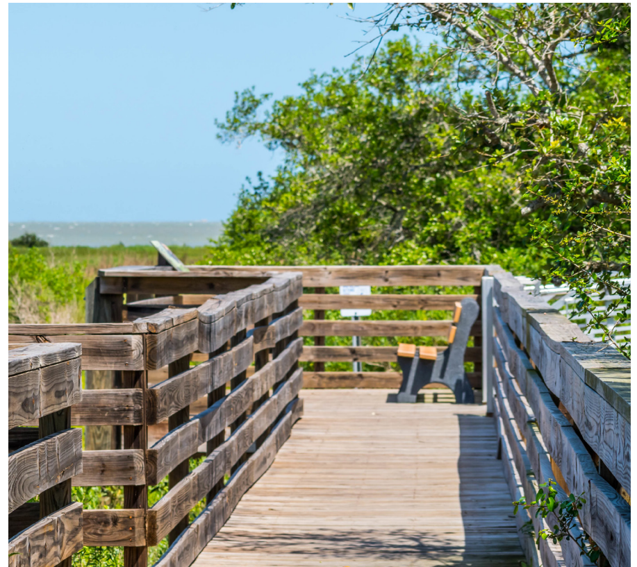
Typical Timber Boardwalk
