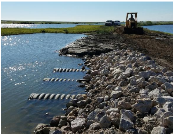
New culverts under levee restore hydrology to marsh.
